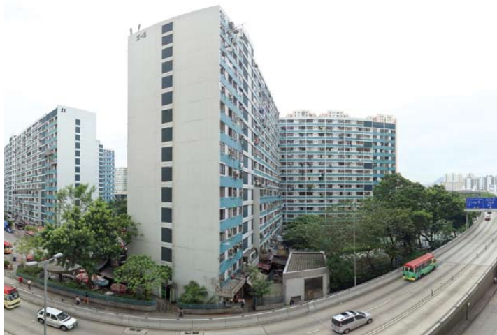
牛頭角下區是「整體重建計劃」中最後一個屋區。 LNTKE is the last estate covered by the Comprehensive Redevelopment Programme.
