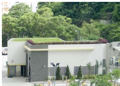
垃圾收集站設於通風良好的位置，而且有一個綠化屋頂。 The refuse collection facility comes with a green roof and is placed in a well-ventilated location.
